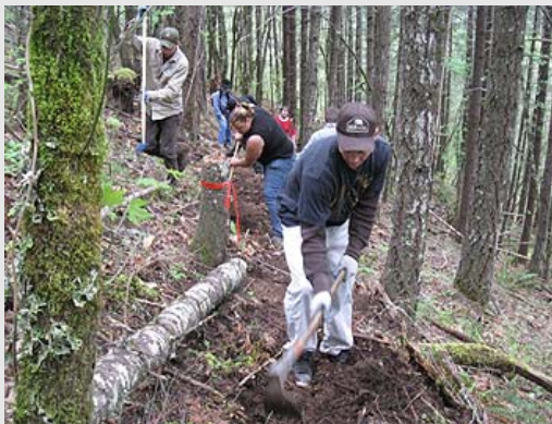
Youth from the Wolf Creek Job Corps construct a new connector trail on the ACCF site, May 2009.
